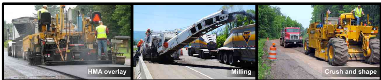
Figure 4: Examples of structural improvement treatments—(from left) HMA overlay on an unmilled pavement, milling asphalt pavement, and pulverization of a road during a crush-and-shape project.
