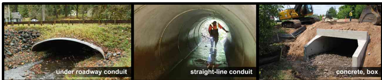
Figure C-2: Examples of culverts. Culverts allow water to pass under the roadway (left), they are straight-line conduits with no intermediate drainage structures (middle), and they come in various materials (left: metal; middle and right: concrete) and shapes (left: arch; middle: round; right: box).
